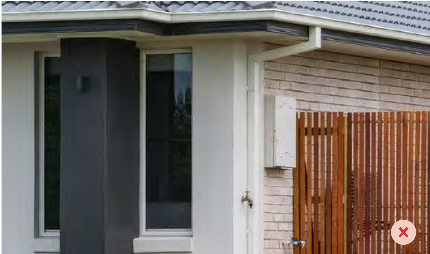
Render not returned to meet the line of the side fence.
